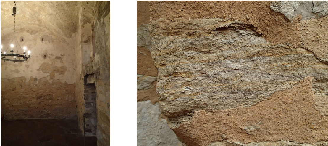
Figure 4: (left) Evidence of rising damp and loss of plaster on the interior wall. (right) Deterioration of stone through delamination
