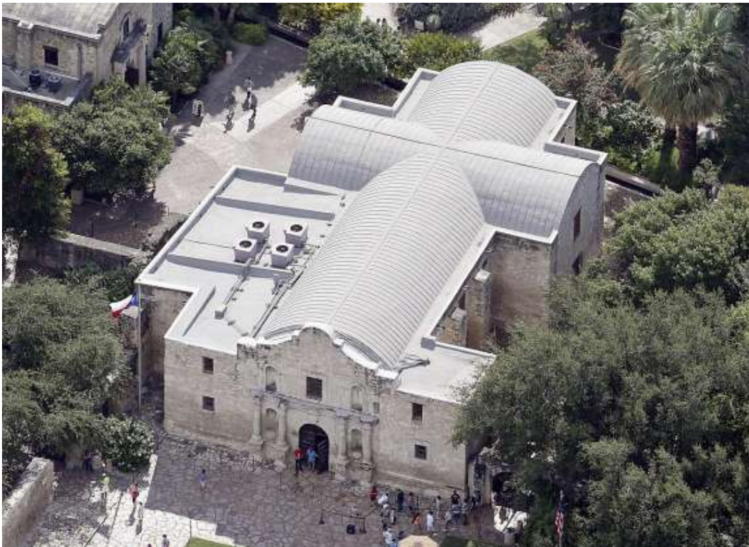
Figure III.3: 2015 Image showing the contemporary lead and concrete roof 3
